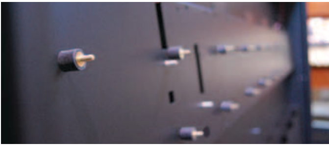
Rubber vibration-isolation mounts
