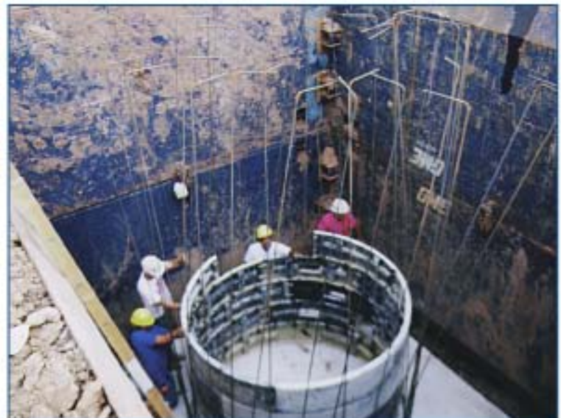
Pit application with stacked shields.
