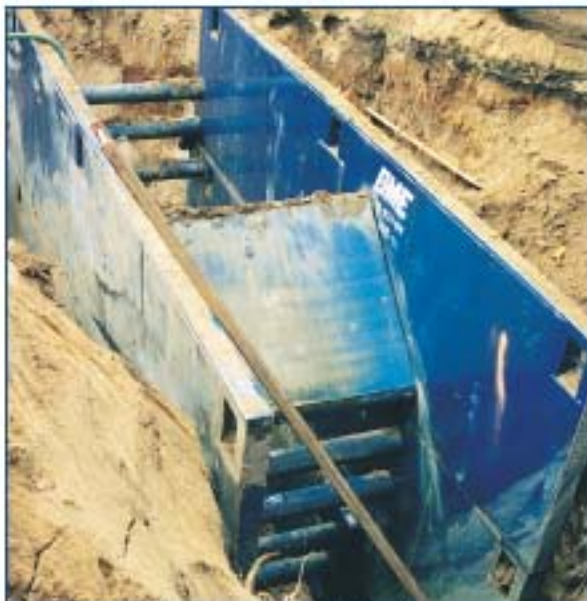
Special shield using a custom bedding slide.
